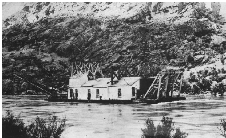
Early 20 th century gold dredge 'Endeavour' working the Molineux
